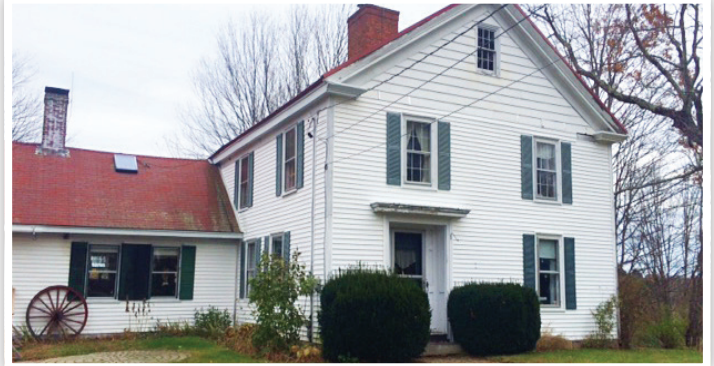
The house today. It has not changed very much in recent years.
